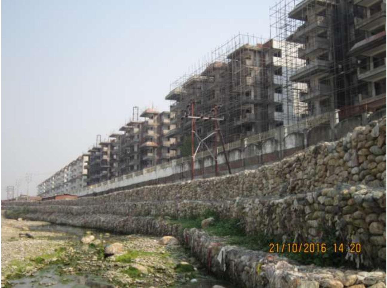
Gabion wall constructed adjacent to north side boundary wall in 31 May 16 to prevent flooding and soil erosion.
