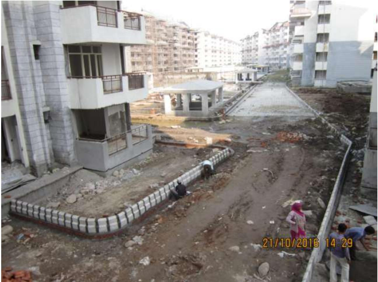
**PROGRESS:** Overall 25% area development over Non-Tower Area upper basement roof has been achieved. Works are like roof top water proofing, filling of earth and laying of fire fighting path are in progress.
