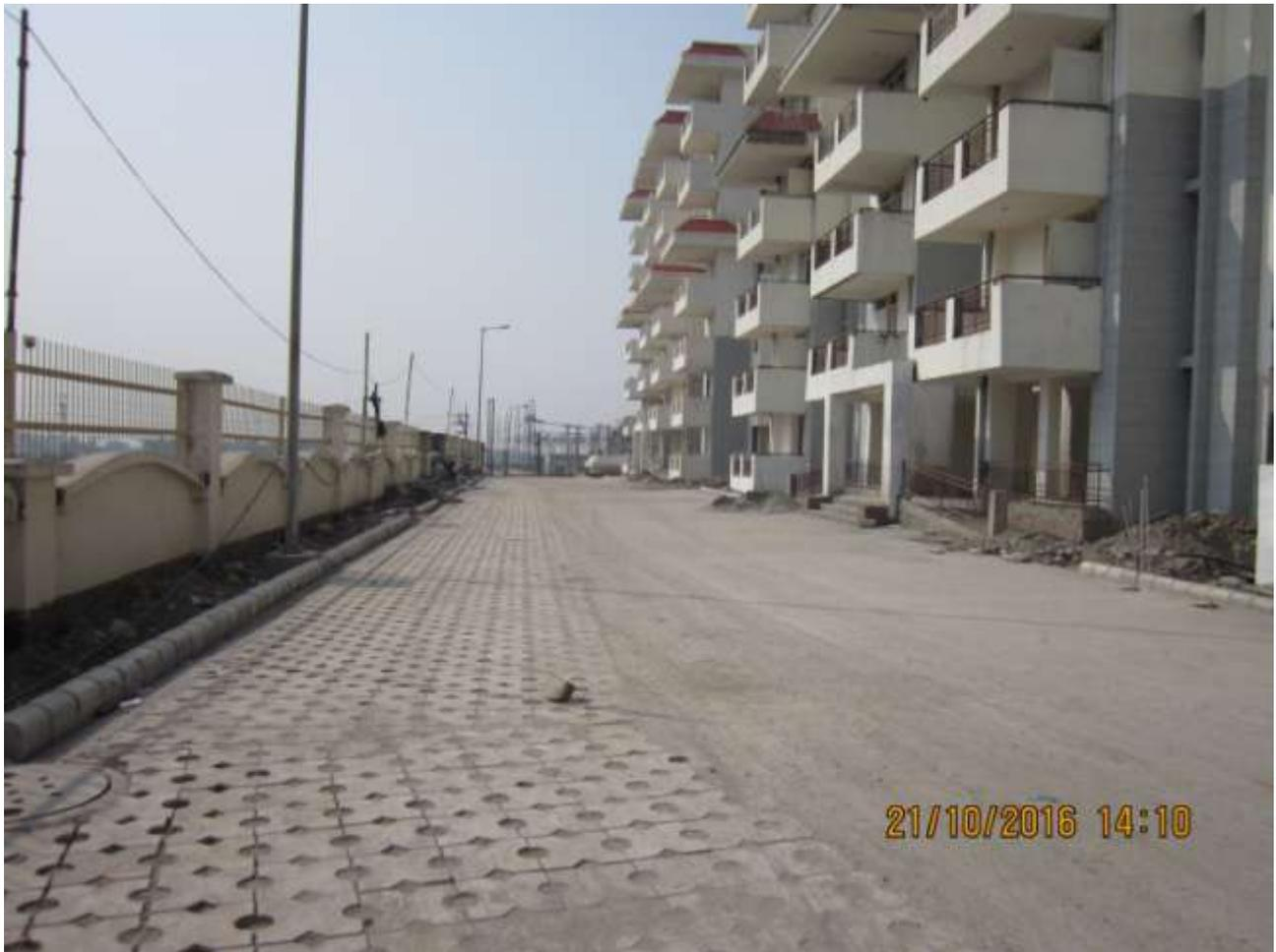
**PROGRESS:** Overall 90% area development work on south side has been achieved. Works are like laying of Concrete road, paver blocks upto gate no. 02, sewer/drain line connected up STP, external fire fighting line, HDPE water line has been completed.
