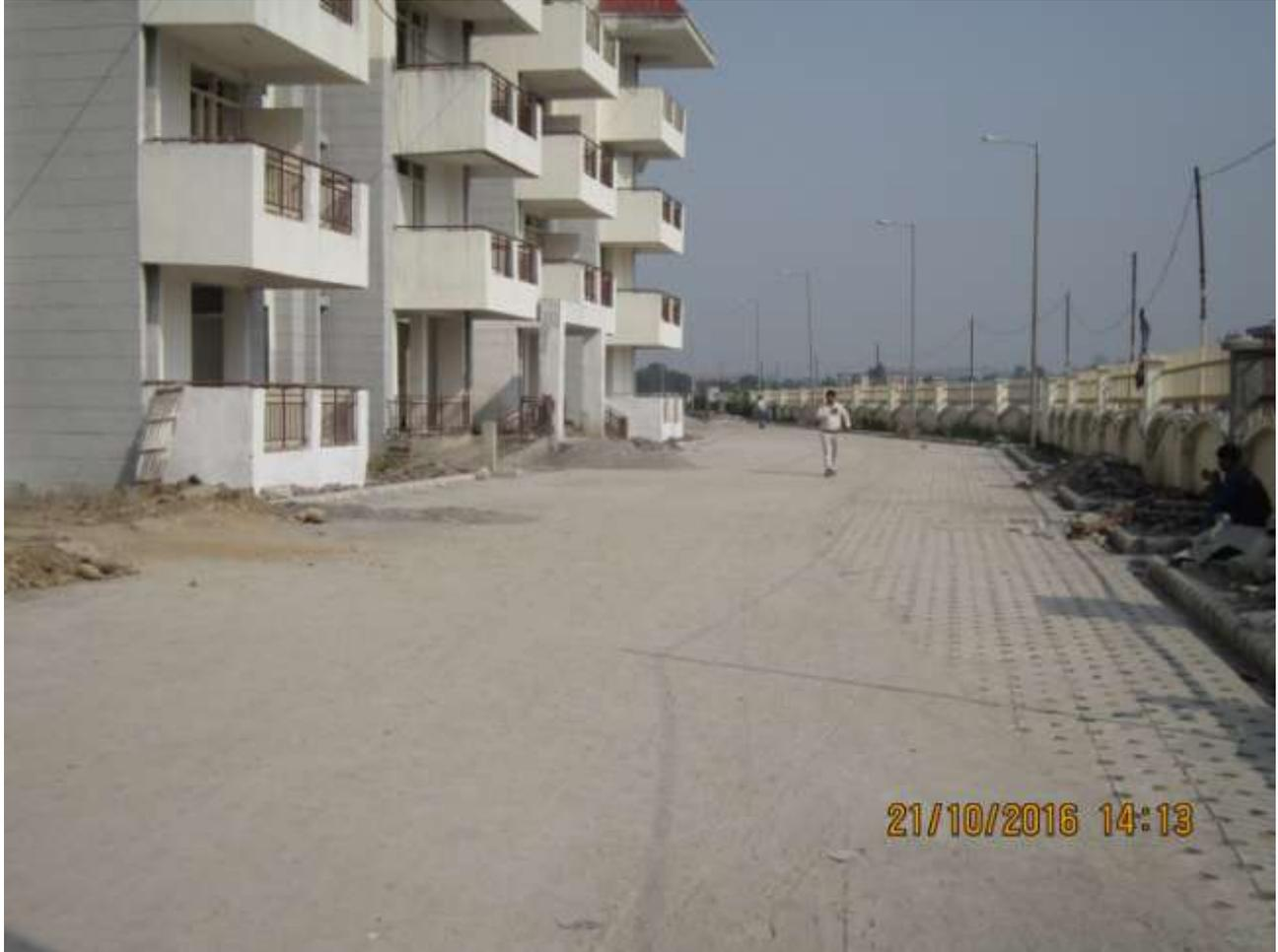
**PROGRESS:** Overall 90% area development work on south side has been achieved. Those works are like laying of CC road, paver block upto gate no. 02, sewer/drain line connected up STP, external fire fighting line, HDPE water line has been completed.
