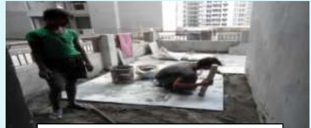
FIXING OF KOTA STONE AT PODIUM
