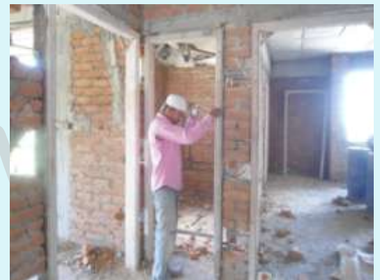
FIXING OF DOOR FRAMES
