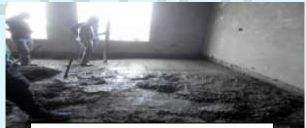
CC FLOORING IN MACHINE ROOM
