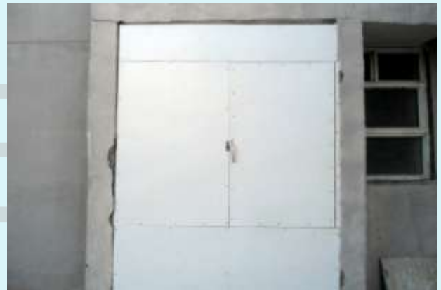
FIXING OF SHUTTER AT PLUMBING SHAFT
