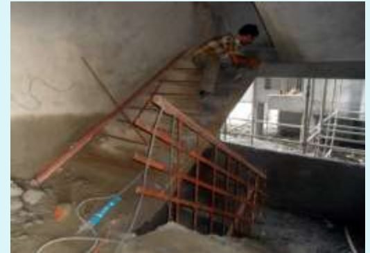
FIXING OF RAILING OF STAIRCASE
