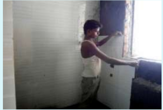
FIXING OF TILES IN TOILET
