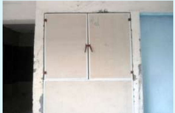
FIXING OF SHUTTER AT ELECTRICAL SHAFT
